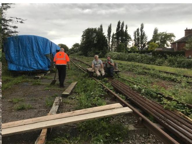
The arrival of the new-to-us rail, apart from extending the siding length, has meant that the temporary short rail sections in use have now been replaced with some of the new stock. A short video recently put on the
