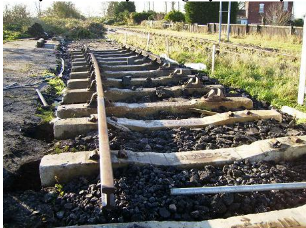
A new siding under construction at Waldersea.
