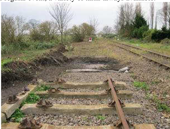
The next stretch of siding under construction.
